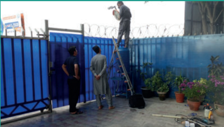
Entrance of the residence redesigned and new security cameras installed
