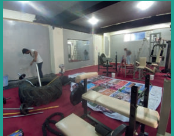
Gym facility renovated with new equipment
